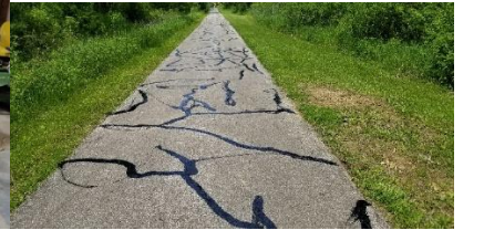
Crack sealing east trail
