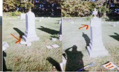
Oakdale Cemetery repairs
